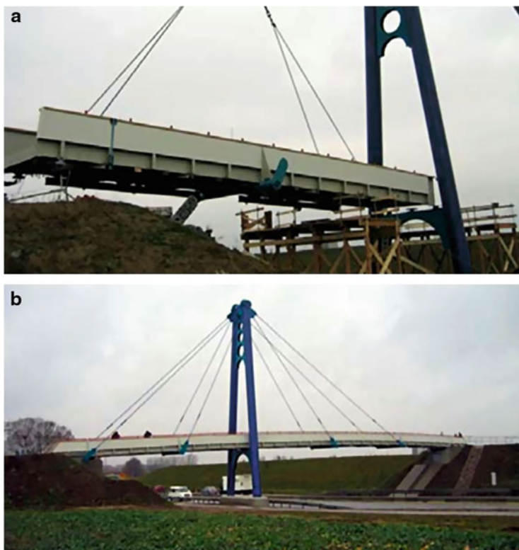
Fig. 16.1 Pedestrian Bridge in Schwerin, Germany. A two-component epoxy structural adhesive was used in this bridge to bond prefabricated elements of GFRP (glass fibre-reinforced polymer composite having an unsaturated polyester resin matrix) constituting the segments used in the bridge deck [4]
