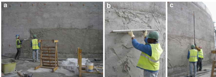
Fig. 2.25 (a) Application of the base coat with spraying device, reference points; (b) pressing and smoothing/levelling the mortar's coat; (c) checking the render's verticality with a reference support [67]
