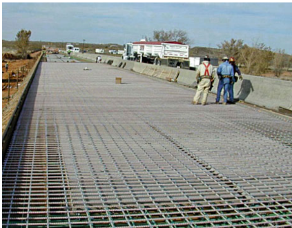
Fig. 11.9 Concrete bridge deck reinforced with GFRP bars
