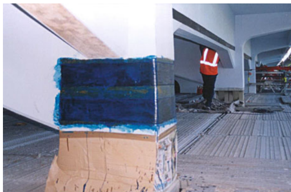
Fig. 11.12 CFRP sheets used in the strengthening of Duarte Pacheco Viaduct
