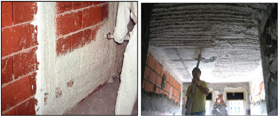
Fig. 3.48 Examples of coating application using spraying devices [27]
