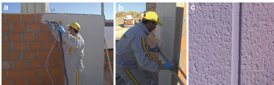
Fig. 2.26 (a) Application of one-coat render by spraying; (b) pressing and levelling with aluminium ruler; (c) final aspect of a mortar joint
