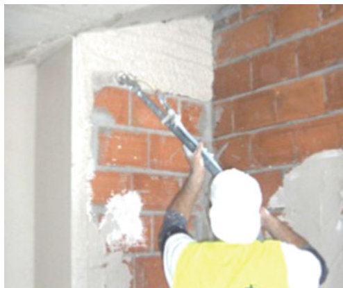
Fig. 3.20 Spraying of the paste in successive horizontal strips [25]
