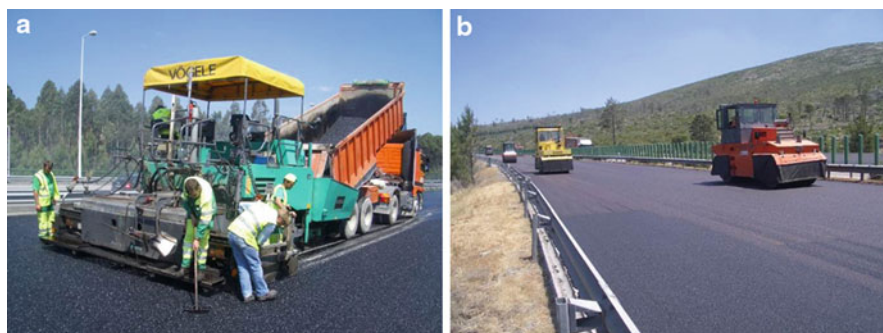
Fig. 5.9 Pavement construction: (a) asphalt paver; (b) rollers operating the bituminous mixture compaction
