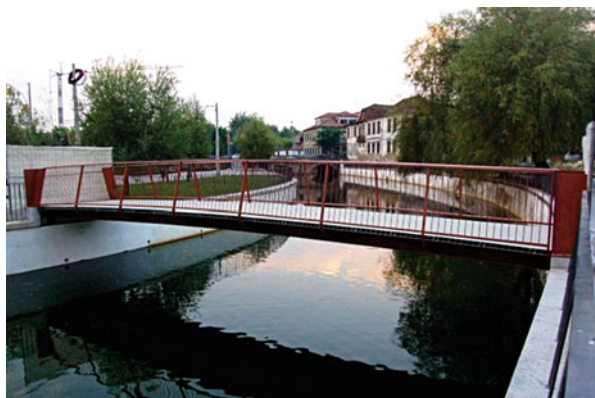
Fig. 11.13 Steel/GFRP hybrid footbridge in Viseu, Portugal
