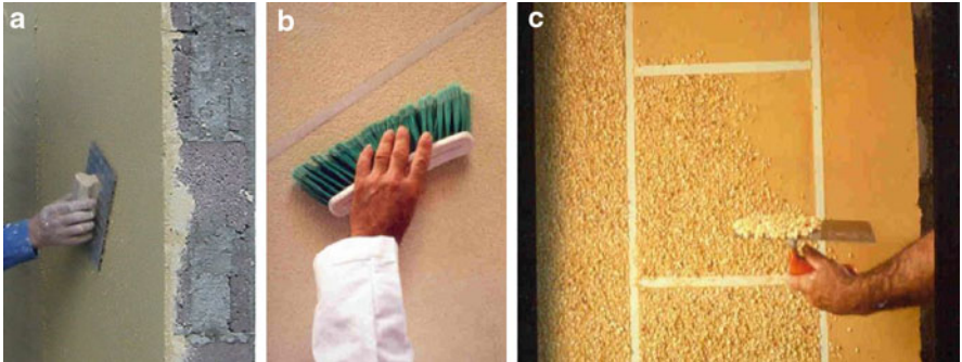
Fig. 2.27 (a) Execution of scraped finish: floating and (b) scrubbing; (c) application of finish in stone in pre-dosed renders [64]
