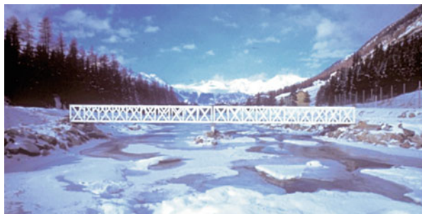
Fig. 11.14 All-FRP Pontresina footbridge [46]
