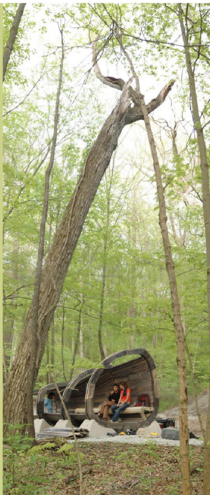
Kevin Klinger, Calibration Channel, 'Digital Exchange', 2006 The Calibration Channel interior is constructed from a series of hybridised timber frames lined with red oak and ash planks.
