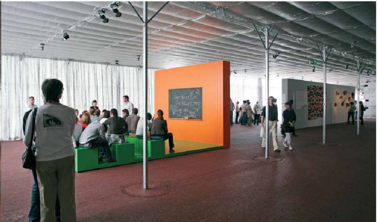
Discreet steel-profile posts, set in a regular rhythm, are the only visible structural elements and plunge directly into the dirt-red bitumen floor. (Artwork: Gerwald Rockenschaub, Klassenzimmer , 2007.)
