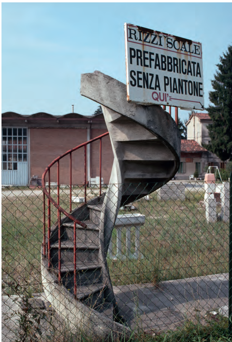
Concrete factory, Vicenza, Italy.
