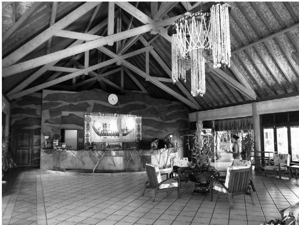
Figure 4.3.10 The reception area is naturally ventilated; stone and tiles are easy to maintain and help in moderating temperatures.
