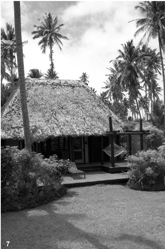
Figures 4.1.7–8 The design of individual guest units is based on traditional Fijian houses. Their high cathedral ceilings, lightweight thatched roofs and generous louvered windows on both long sides ensure an excellent thermal environment even without air-conditioning.
