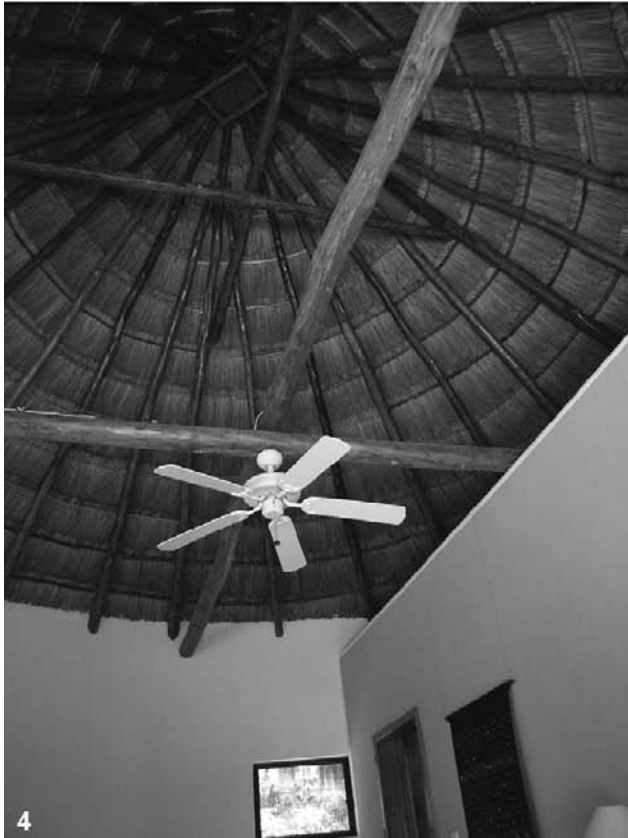
Figures 4.6.4–5 Second-storey units benefit from high cathedral ceilings allowing hot air to rise under the roof; ground floor units have their thermal environment shaped by the openness of the plan and staying permanently in the ‘shade’ of the upper floor.
