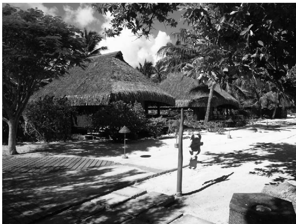
Figure 4.3.4 The architecture of all bungalows at the resort relates to local traditions not only in form and colour but also choice of materials, with prominent pandanus thatch and extensive use of timber.
