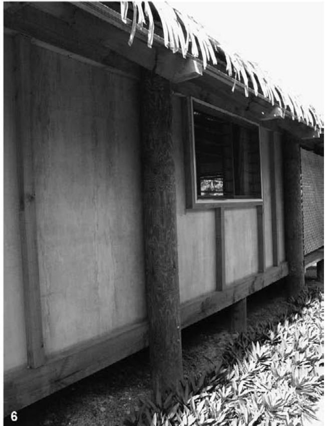
Figures 4.4.2.5–6 Large shaded verandas (Are Tamanu) and single-skin plywood walls (Muri Beach Hideaway) ensure a thermal environment within the comfort range during most of the year.
