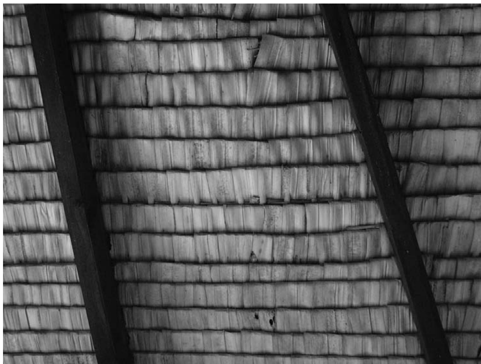
Figure 4.3.6 Detail of roof thatch seen from the interior.
