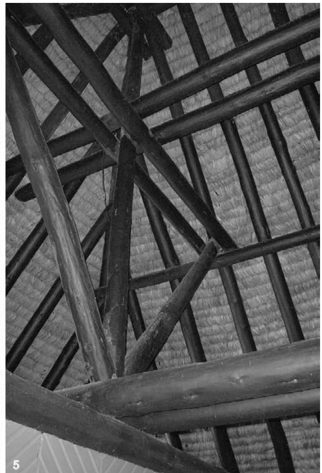
Figures 4.1.4–5 Thatched roof over the dining area; constructed, maintained and repaired by the local craftspeople.
