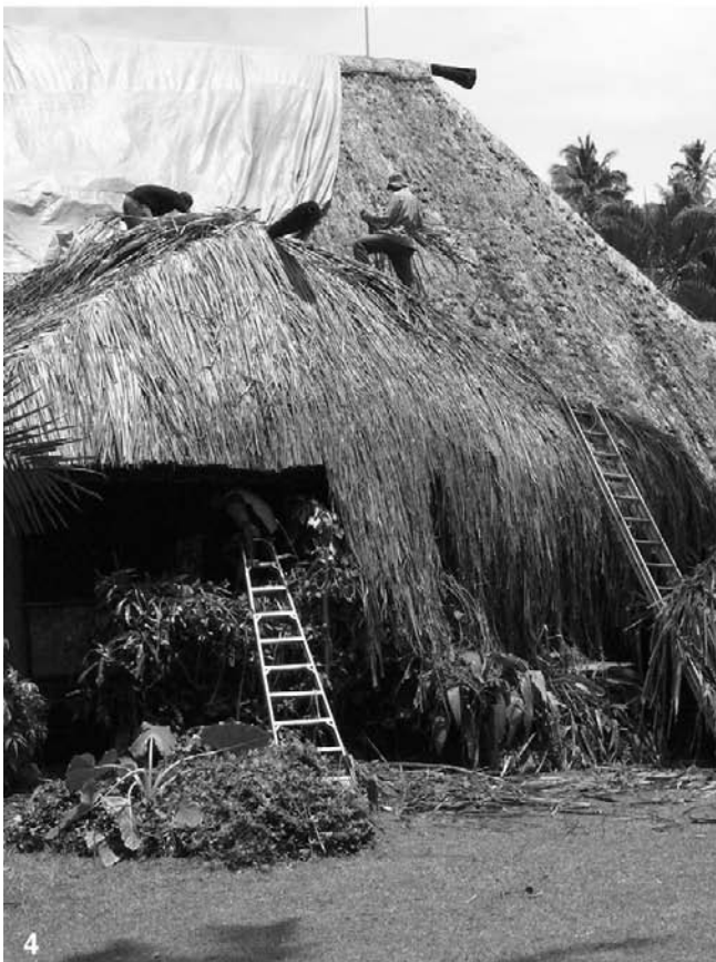
Figures 4.1.4–5 Thatched roof over the dining area; constructed, maintained and repaired by the local craftspeople.
