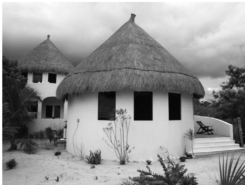
Figure 4.6.1 Balamku Inn comprises guest units housed in single- and double-storey buildings.
