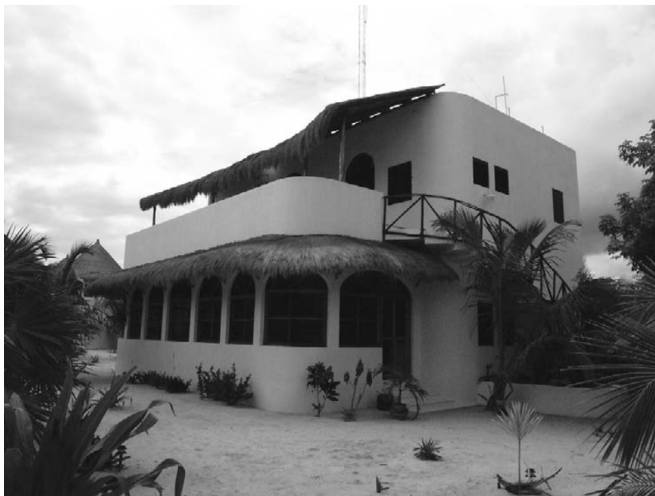
Figure 4.6.3 The largest building contains the reception, resort dining room and kitchen, with the office and owner/operator accommodation on the upper floor.
