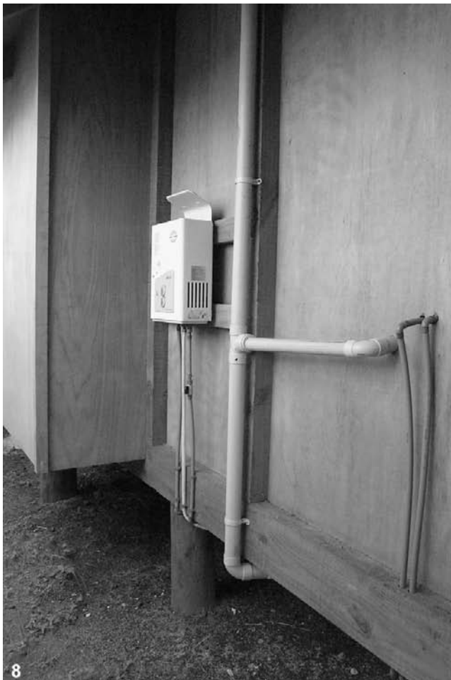
Figures 4.2.8–9 Instantaneous gas heaters were found to be the cheapest and most reliable means of water heating at the Muri Beach Hideaway; energy savings are achieved by using solar-powered lighting of the site.
