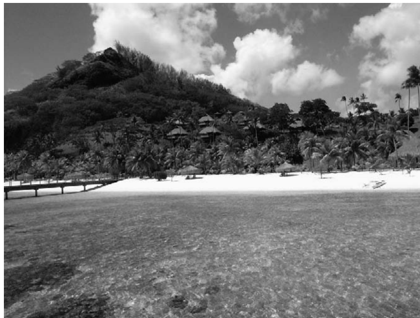
Figure 4.4.6 The 600 m long artificial beach was built with sand dredged from the atoll's shipping channel.
