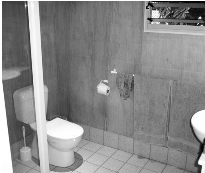
Figure 4.2.7 High quality plywood walls do not require finishing on the inside and their maintenance is inexpensive and easy (Muri Beach Hideaway).
