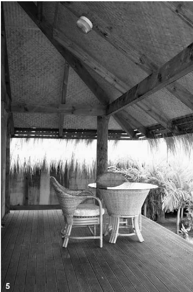
Figures 4.4.2.5–6 Large shaded verandas (Are Tamanu) and single-skin plywood walls (Muri Beach Hideaway) ensure a thermal environment within the comfort range during most of the year.
