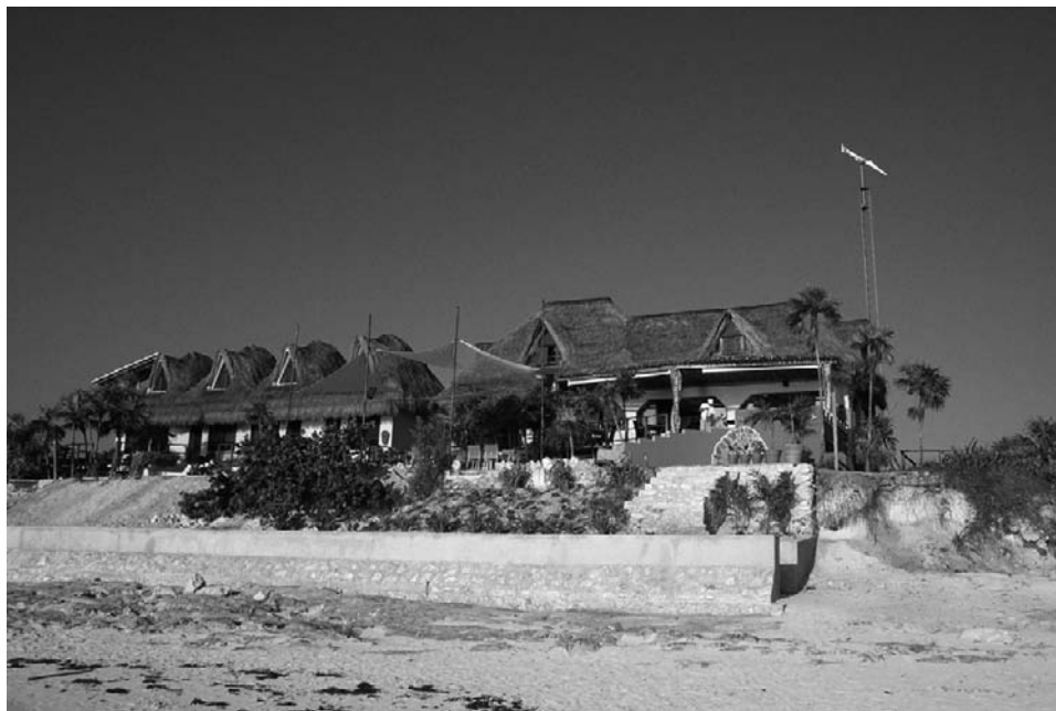
Figure 4.5.1 General view of the Mezzanine from the water edge; retaining wall protecting the escarpment against storm surges is clearly visible as are wind turbine and solar panels.
