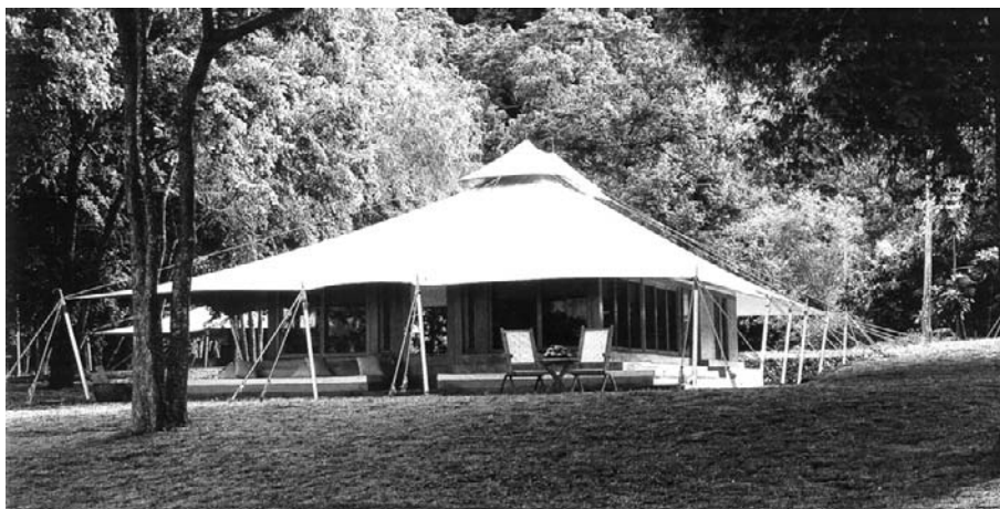
Figure 3.16 A parasol roof on a guest unit at Amanwana Resort, Indonesia.
