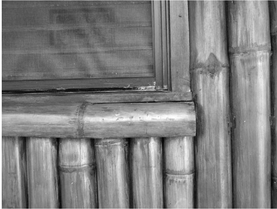
Figure 4.3.5 Detail of bamboo wall cladding.
