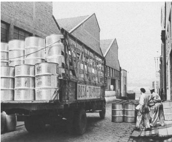
Lina Bo Bardi, SESC-Pompéia: site as factory before construction.
