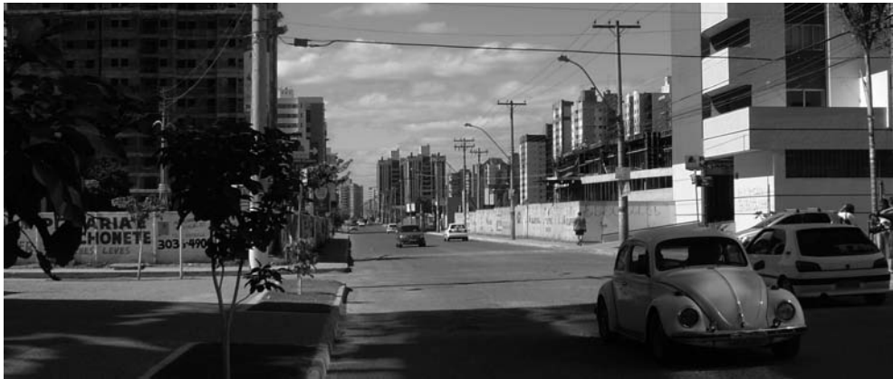
Águas Claras, central avenue under construction, 2006.
