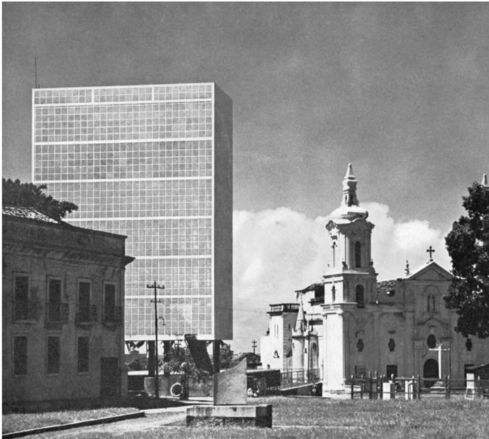
Luis Nunes, Olinda water tower, 1937. Reproduced in Brazil Builds .
