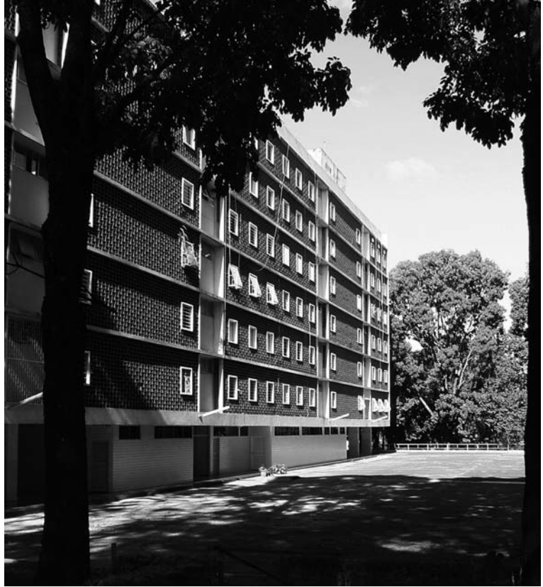
South wing superquadra blocks, Brasília, c. 1957–60.
