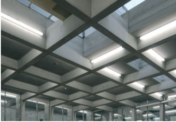
The coffered concrete ceiling of the central hall. Light is admitted from above. The new chapel, which sits atop this large space, acts as a flue for the natural ventilation strategy.
