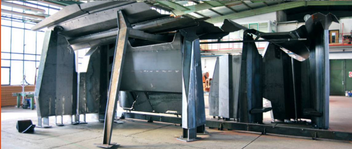
View from the southeast corner, near to completion.
