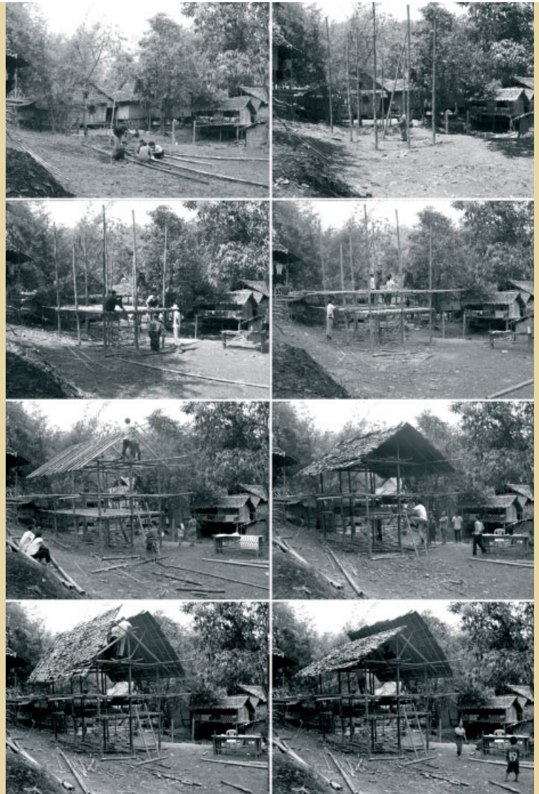
Time lapse view of the prototype construction at the Mae La refugee camp. Local craftsmen adapted the students' proposal and the two groups collaborated to construct a single-family house for performance assessment.
