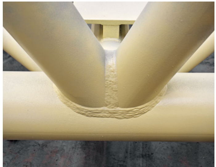
A primer is applied over the metalizing to provide a base for the final paint coating. The selection of the primer will depend on the requirements of the final paint finish or coating. The welds have been neatly done and left exposed at the panel points of the truss.
