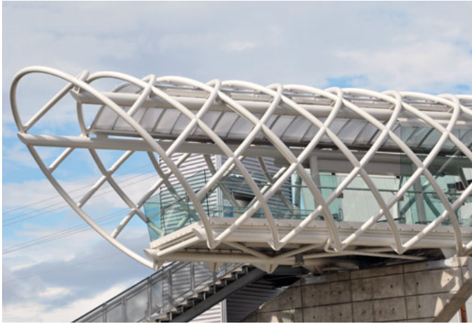
The pedestrian bridge at the Museum of Flight in Seattle, WA, USA, designed by SRG Partnership Inc. and Magnusson Klemencic Associates, is served by AESS 3 type steel due to the close view maintained even to the height of the bridge. The added complexity of the curvature and welding of the round HSS "hoops" adds to the cost of this structure.
