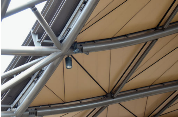
The exposed steel roof of the Southern Cross Rail Station in Melbourne, Australia, designed by Grimshaw Architects, is finished in a medium grey, which is excellent at masking evidence of grime.
