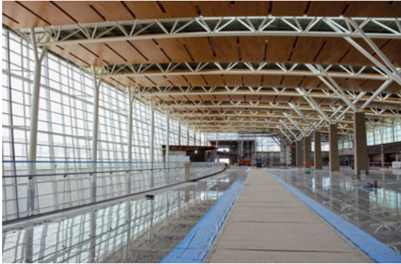
The International Terminal at Calgary International Airport in Calgary, AB, Canada, designed by DIALOG, uses AESS 2 standards for the trusses that span the hall. They are fabricated from a combination of round and square HSS. The major lengths of the trusses are achieved using fully welded connections with no weld remediation. The columns and struts are AESS 3 due to their proximity and specific connection detailing.
