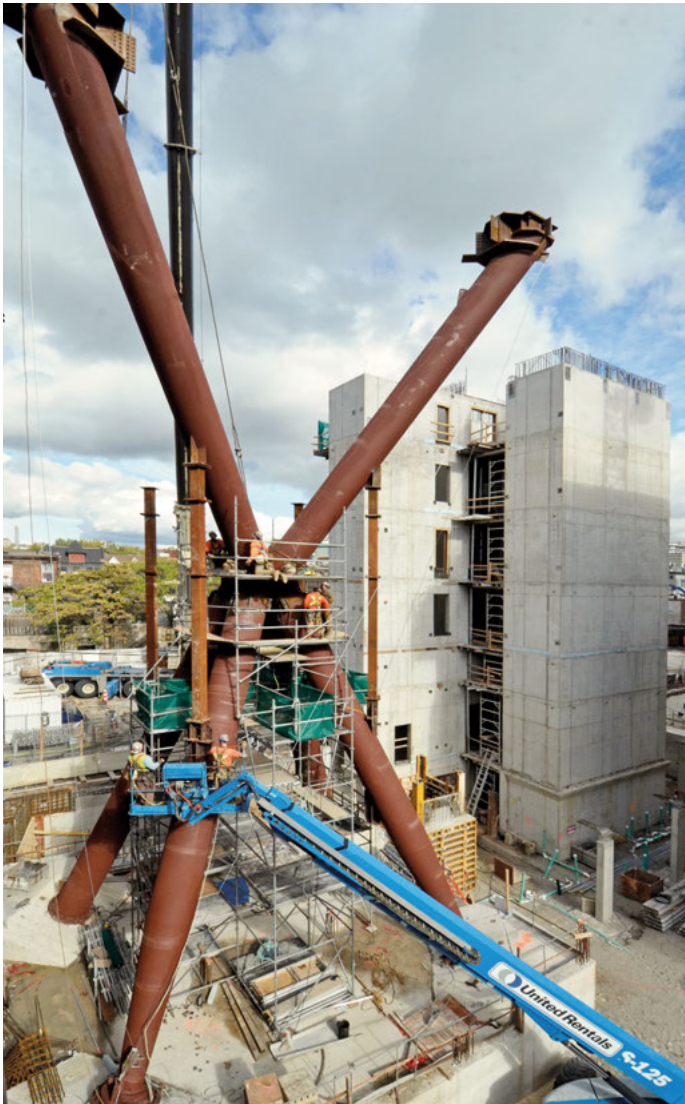
Restricted site access, a densely built-up site and the angled steel supports on QRC West in Toronto, ON, designed by & Co Architects, make this a logistical and sequencing challenge. A large crane to the back of the site lifts the steel leg. A smaller lift is required to access the connections to complete the temporary bolting. Fabrication and erection by Walters Inc.
