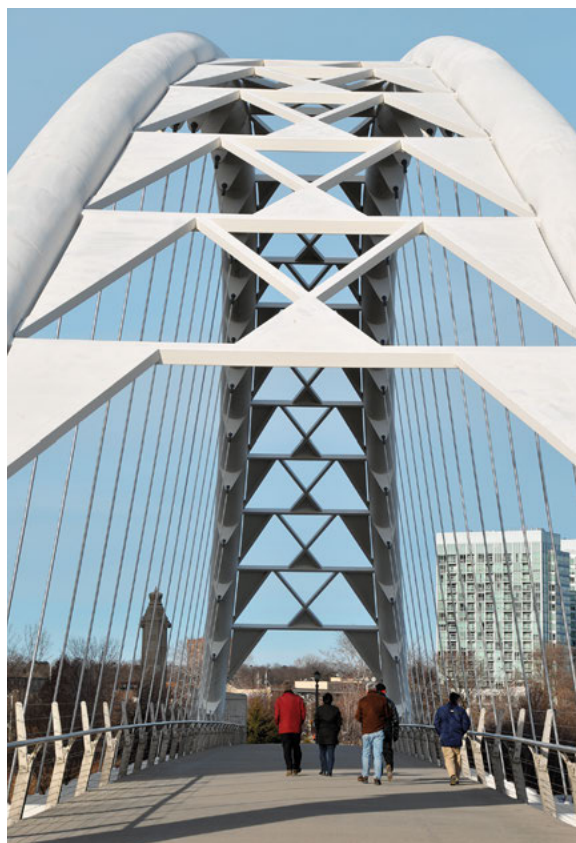
The Humber River Bridge in Toronto, ON, Canada, designed by Montgomery and Sisam Architects, uses large-diameter, helically welded tubes for the main spanning sections of the arch.
