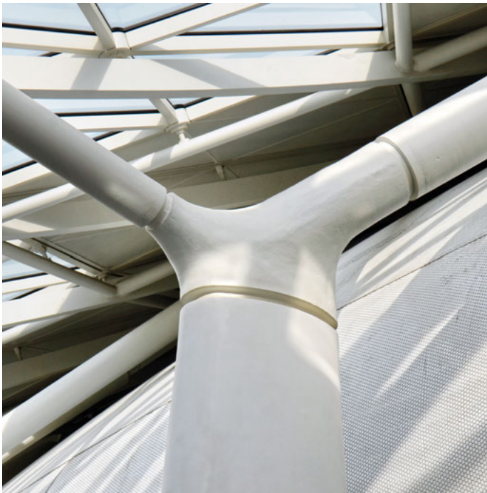
The World Financial Center entry pavilion uses custom-bent steel to create this pair of diagrid column supports. The connections are all welded, incurring additional expense and challenges on the site to prepare scaffolding to carry out the work. The expectation was that the numerous on-site welds would be remediated to the same high quality as those done in the shop.
