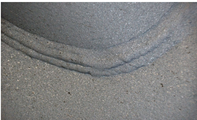
A close view of the surface of a welded connection after the application of metalizing.
