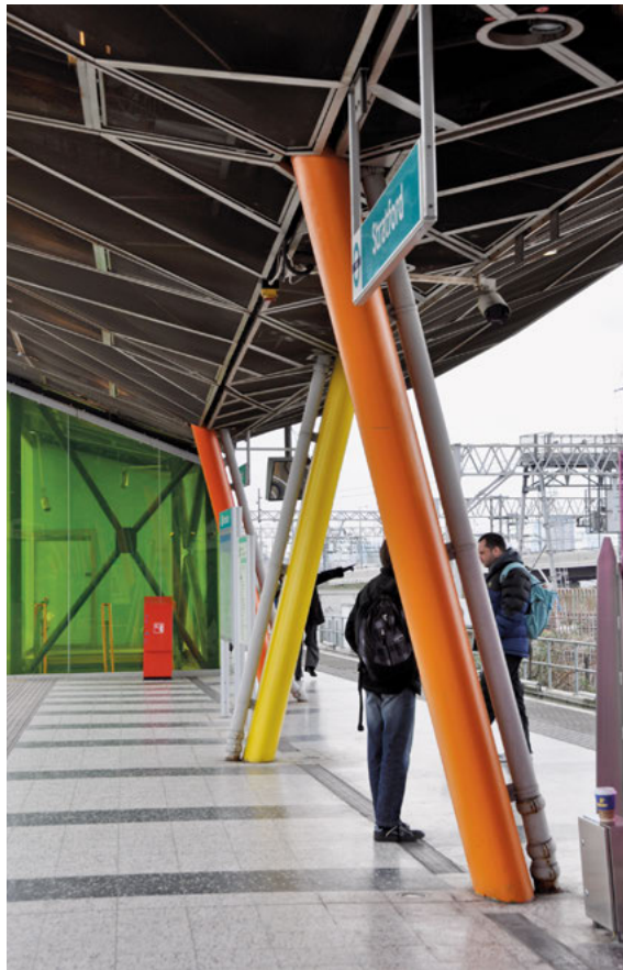
Sloped elliptical tubes are used at the Stratford DLR Station in London, England, designed by SMC Alsop Architects, to provide architectural interest to the simple structure of the station. The end connections are hidden to focus attention on the shape of the members, which are also highlighted by the use of bright colors.
