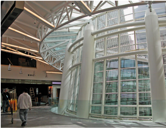
Intumescent coating is used to allow the exposure of the steel in the atrium of the Bloomberg Building in New York City, NY, USA, designed by Pelli Clarke Pelli Architects.
