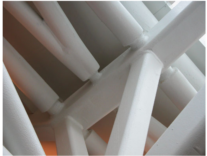
The detailing of the Bloomberg Building has been designed with the thickness and finish of the coating in mind. The details are simple and the reveals around the connections are designed to add evidence of form to the connections. The texture of the finish is evident. There would be no benefit in contouring and blending the welds.
