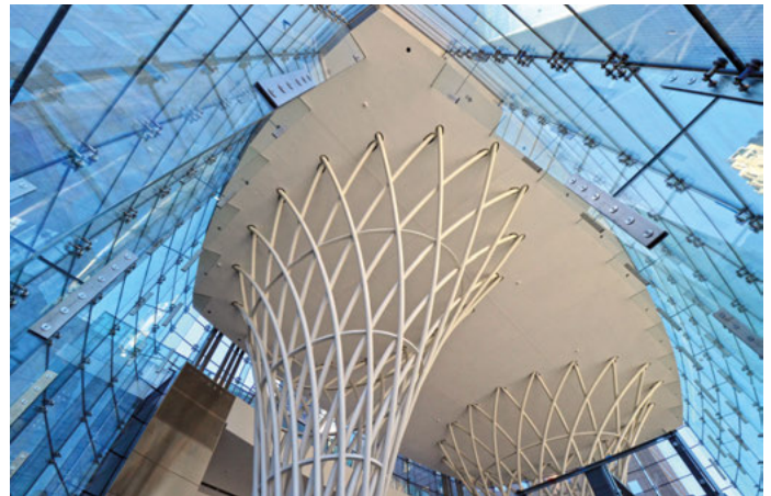
The World Financial Center entry pavilion uses custom-bent steel to create this pair of diagrid column supports. The connections are all welded, incurring additional expense and challenges on the site to prepare scaffolding to carry out the work. The expectation was that the numerous on-site welds would be remediated to the same high quality as those done in the shop.
