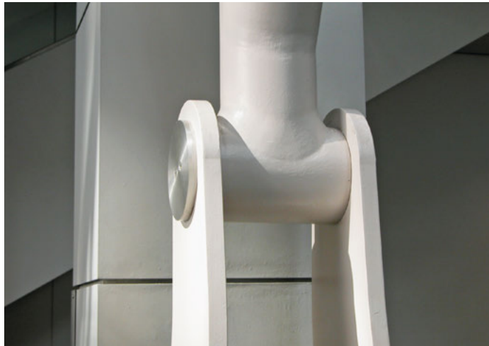
This welded tube-to-tube detail at the Rose Center for Earth and Space has the welds ground and filled, creating an extremely smooth transition. This detail is located near eye level and truly required such remediation to maintain the sculptural feel of the design.
