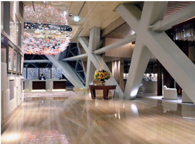
Capital Gate in Abu Dhabi, UAE, designed by RMJM Architects, uses an intumescent fire protection strategy to allow full exposure of its custom-fabricated diagrid frame.
