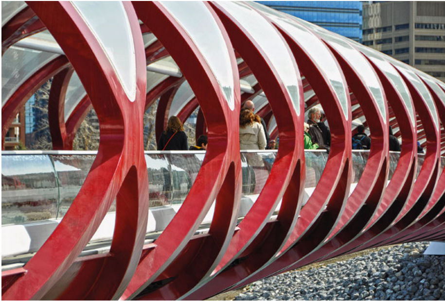
The pedestrian Peace Bridge in Calgary, AB, Canada, designed by Santiago Calatrava, has used a high degree of brake forming, welding, grinding and filling to create this tubular shape. A structure like this would sit at the extreme high end of AESS 4 expectations and cost premium.
