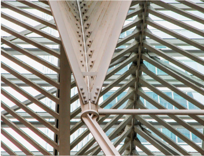
The high-end AESS detailing of Brookfield Place in Toronto, ON, Canada, designed by Santiago Calatrava, 1996, was long looked at as a quality benchmark for all AESS detailing. Yet even in this project, the nature of the fabrication and joints is different at the base and at the skylight support system. Welding is used at the lower levels where a continuous, smooth finish is desired; bolting is used at the higher levels where visual access is more limited.
