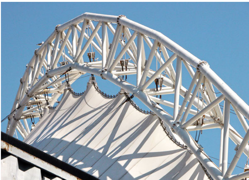
The triangular arched truss that supports the fabric roof of the Bank of America Pavilion in Boston, MA, USA, designed by A.Form Architecture pc, would be classed as AESS 2. It makes use of unremediated welded connections for the tube-to-tube connections within the truss. The truss segments are bolted together. The curved shape is achieved through the use of straight segments, simplifying fabrication. This works as a factor of the scale of the building.
