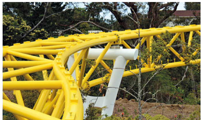
The pedestrian bridge (here under construction) is given final paint coatings to provide the architectural finish.
