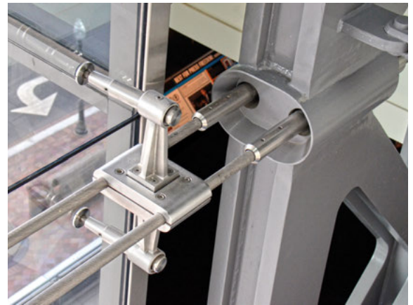
The Newseum in Washington, DC, USA, designed by Ennead Architects with Leslie E. Robertson Associates, makes fairly exclusively uses specialty plate steel for the vertical trusses. The sharp edges and clean lines are characteristically AESS 4. Crisp edges require more care in the application of coatings to ensure good multi-coat coverage at the corners. This truss is located away from danger of chipping due to pedestrian traffic. The extra care and expense in this level of fabrication is warranted as the structure is visible at very close range. It also must coordinate its tolerances with cable and spider glazing systems.
