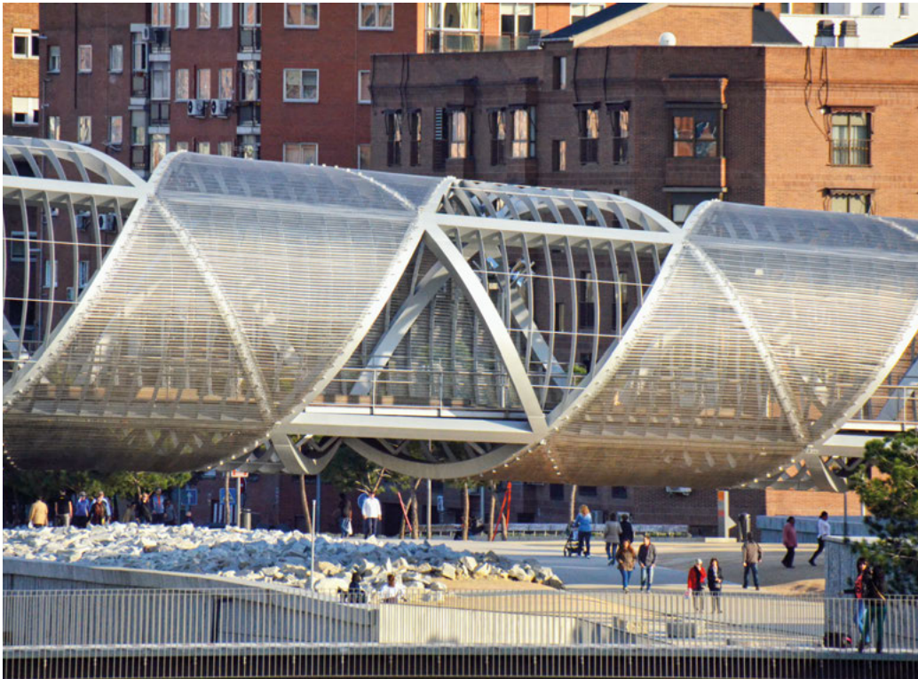
The Arganzuela Bridge in Madrid, Spain, designed by Dominique Perrault, is able to use the scale of the structure to keep the detailing of the welded connections of the curved box sections to AESS 3 standards. The connections within the members use either unremediated welds or bolts.
