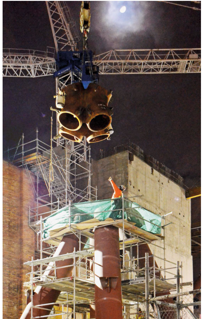
Often streets must be closed off from traffic in order to provide better access to the site for the erection of temporary cranes that complete significant lifts. As this delta frame for QRC West is located directly adjacent to a fairly narrow street, the work had to be scheduled after 8pm to limit the impact on traffic. Night work is more difficult and costly for obvious reasons. Casting designed by CastConnex.
