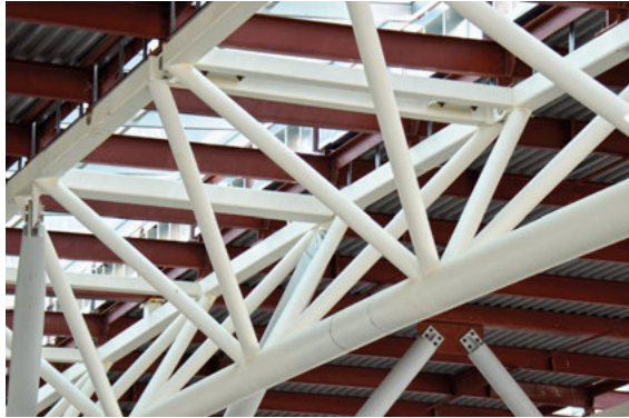
A closer view of the truss shows that a variety of sizes of HSS have been used, dimensioned to suit the loading as well as to allow for ease of welded connections between members. Pin, hidden and discreet connections have been used to join the segments of the truss. Fabrication and erection by Supermétal.
